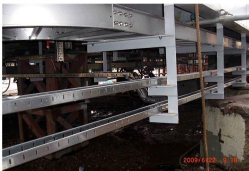
Stainless Steel Cable & Ladder Tray coated with FLEX COTE
